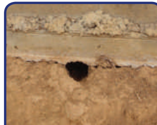
Foundation Burrowing and Damage.
